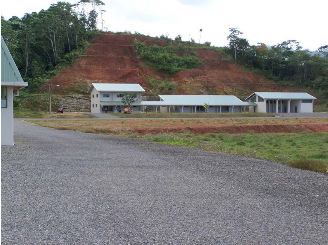
Naboro Landfill Administration Facilities
